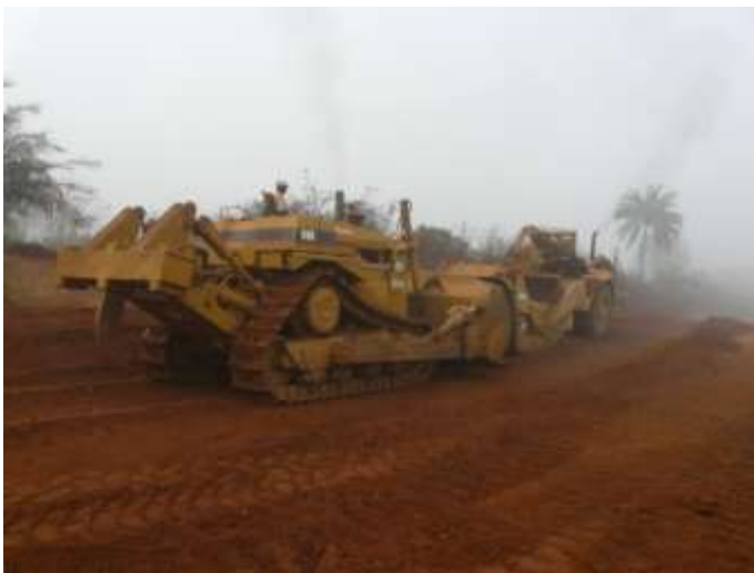
Push and Pull with dozer and scrapper
