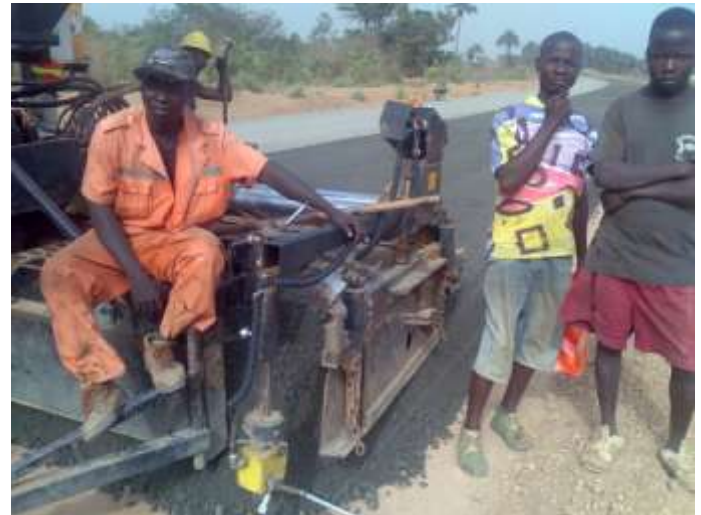
Base Course, built-in with finisher
